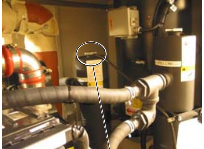
Engine Coolant System Cap
